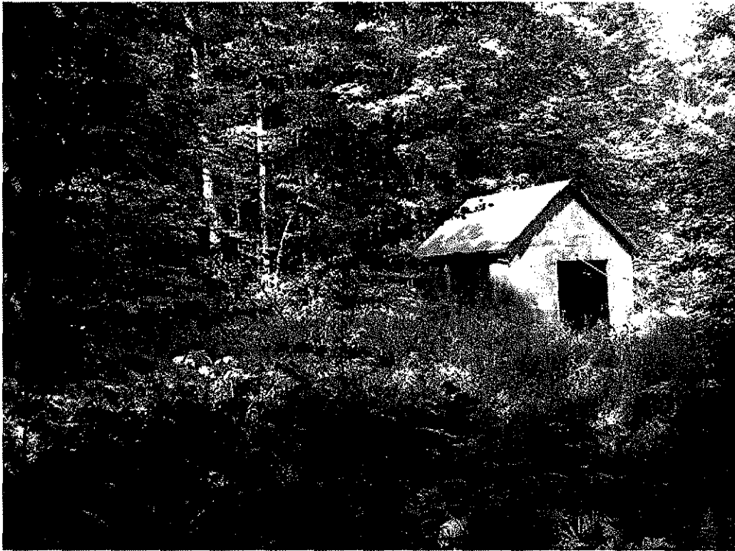
Duhring Powerhouse. Note the pink flagging on the left side of the photo. This is the center-line that will take the access road next to the powerhouse.
