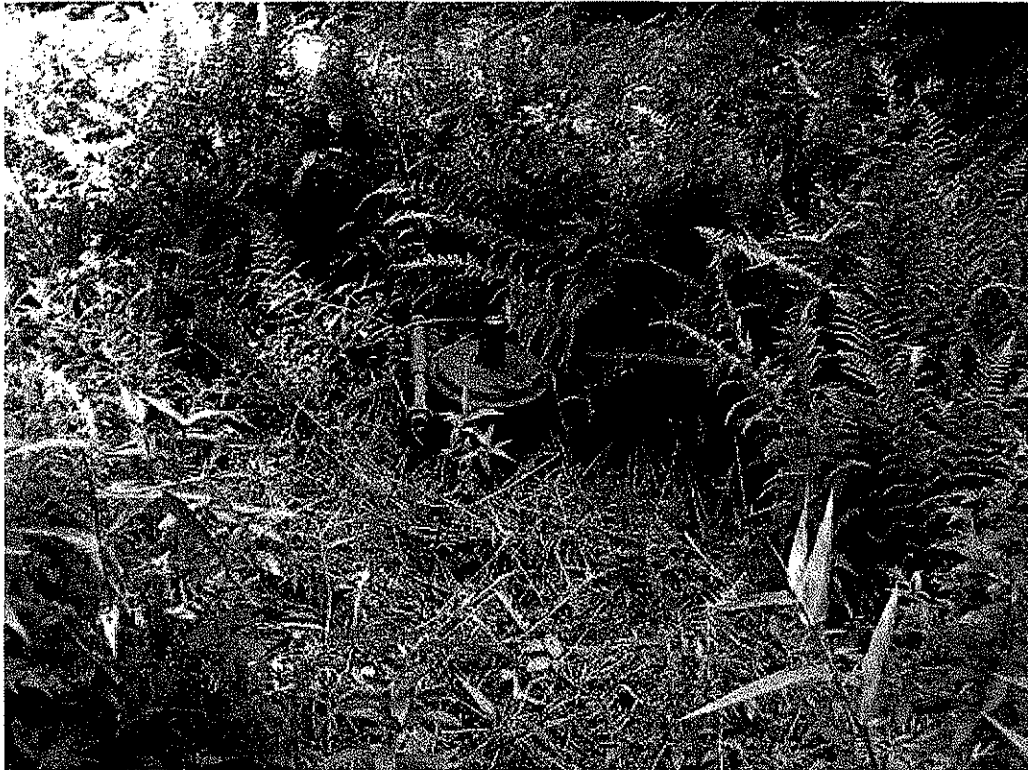
Duhring Powerhouse. Equipment and pipes directly in front of the powerhouse. Purpose is unknown.
